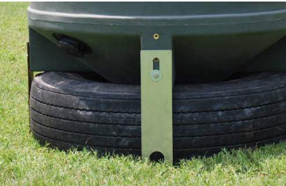
Step 3: Attach tire brackets. (8) Bolt (8) LG Washer
