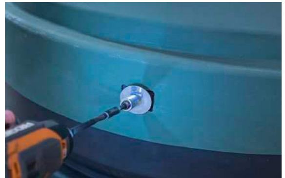
Step 4: Attach dome to base.
