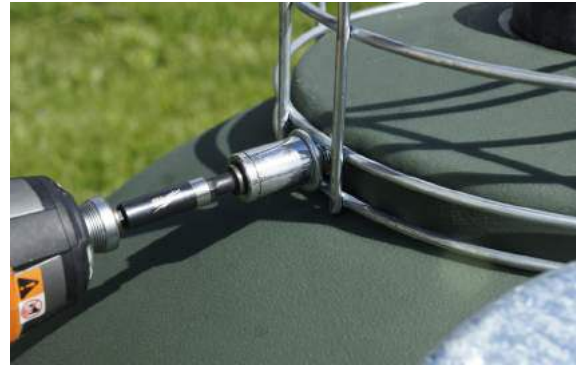
Step 6: Bolt cage to unit.
