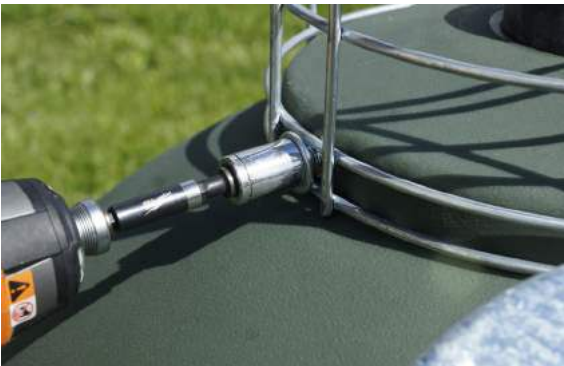
Step 5: Bolt cage to unit.
