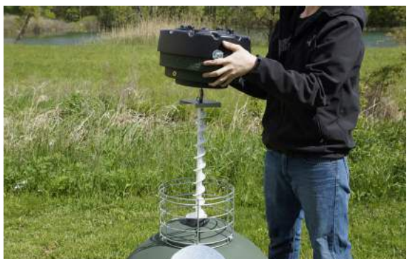
Step 8: Place powerhead on top of cage.
