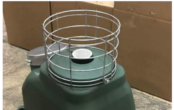
Step 6: Bolt cage to unit.
