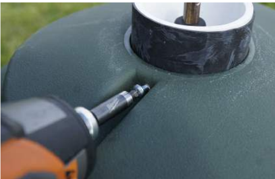
Step 5: Place PVC in hole and attach.
