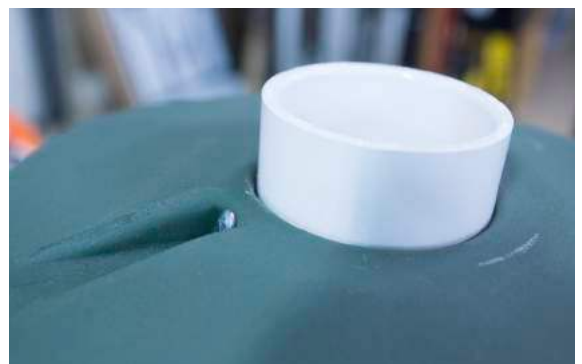
Step 8: Place PVC in hole and attach.
