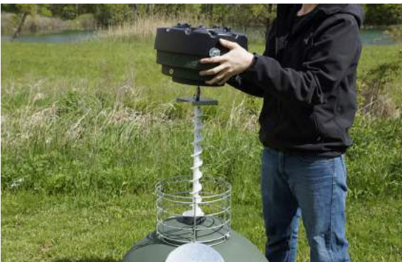
Step 13: Place powerhead on top of cage.
