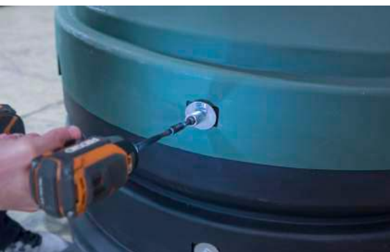
Step 7: Attach dome to extension ring.
